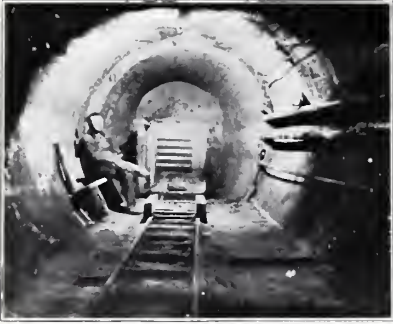
AIR-LOCK—NEW WATERWORKS TUNNEL
